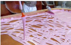
Applying J-Core to the hardtop shell
