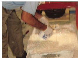
APPLY 60% OF LAMLIGHT over one or two continuous strand glass mats.
